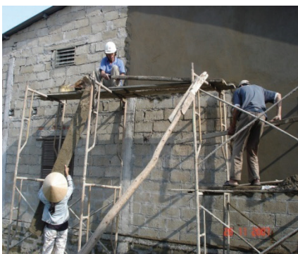
Builders (men and women working together)
